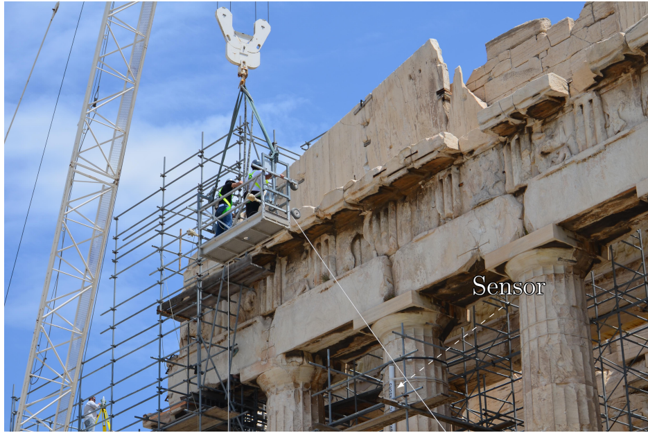
Figure 2.3: Fiber optic sensors are being used for SHM of the Parthenon in Athens, Greece, during renovation. Photo by Lee A. Wymore, used with permission from CRD Group.
