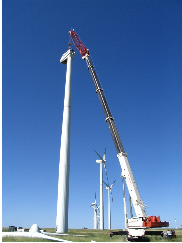
Figure 2.8: Installing a gearbox. Photo by Jeroen van Dam, NREL 19257.
