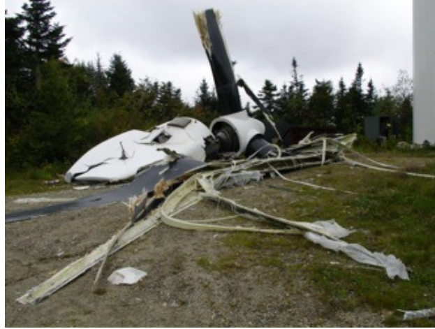
Figure 2.4: Wind turbine failure from high winds shortly after a blade was repaired. Photo by Green Mountain Power, NREL 16713.
